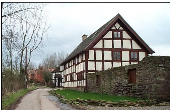
Timber framed houses at Byford
