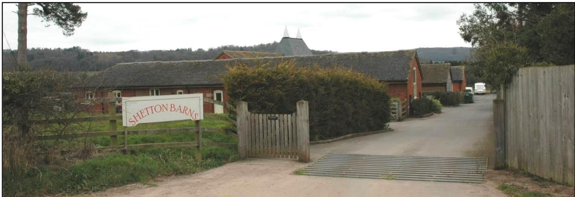
Shetton barn conversions at Mansell Gamage
